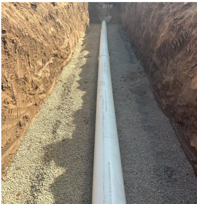
Figure 2: Sewer Gravity Mains laid
